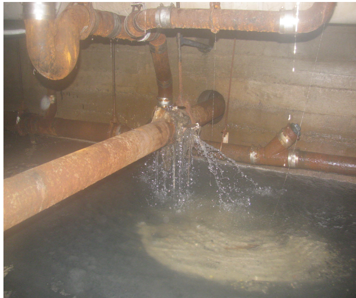
Figure 4 – Example of leaking pipes under prison. Photo: DVI, date unknown.
