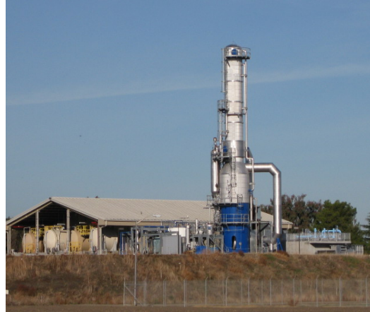
Figure 6 – $32 million non-functioning reverse osmosis water treatment plant. Photo: OIG, November 2010.
