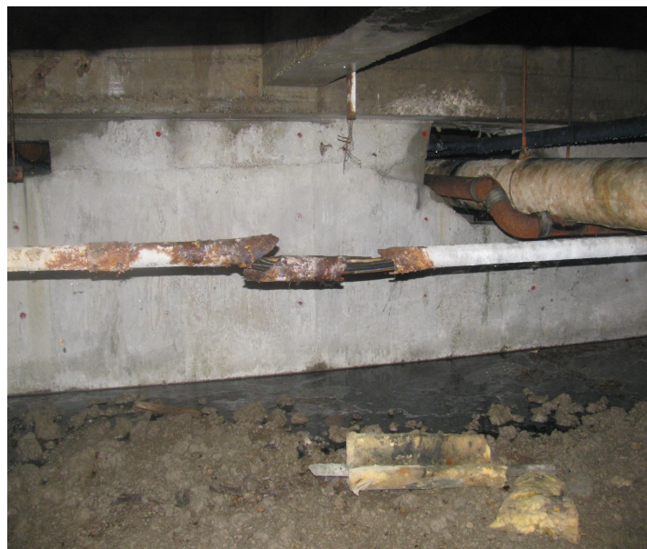
Figure 5 – Example of decaying electrical casing under the prison. Photo: DVI, date unknown.
