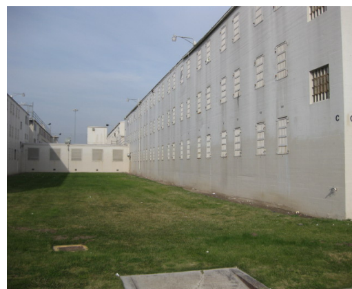
Figure 7 – Example of clean area under exterior inmate windows. Photo: OIG, November 2010.
